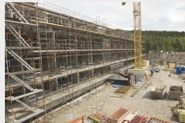
Årvollbrinken housing project in Oslo
